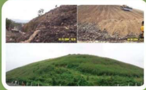
REHABILITATION & CLOSURE OF OPEN DUMPSITE
